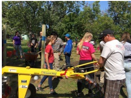
Installing posts for the new fence
