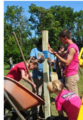
Birmingham 1st Youth Installing a Fence Post on Jane Ave
