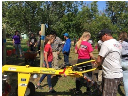
Installing posts for the new fence
