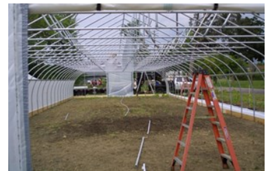
A "High Tunnel" or "Hoop House" is constructed with heavy poly over steel hoops to extend the growing seasons
